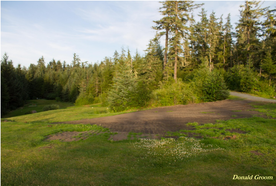
Pictured above is the current construction area on fairway #3.
