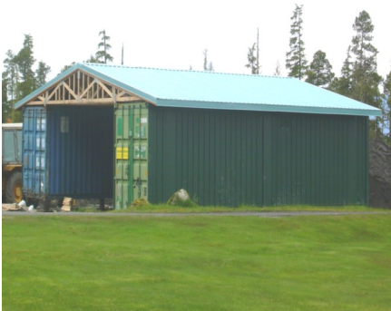
Covered motor cart parking garage. Stalls available for $100/year.
